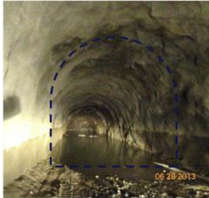
a. Relatively good quality tunnel contour (Upper Tamakoshi Project, Nepal)
